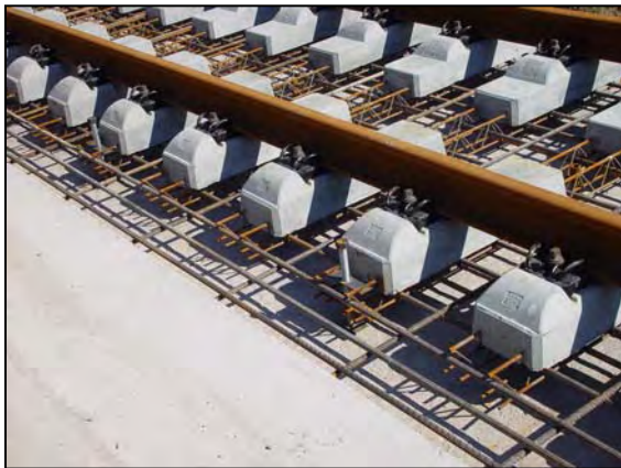
Rheda 2000 Track before infill of concrete
