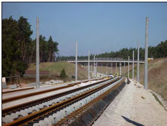
Rheda 2000 Track on embankment during construction
