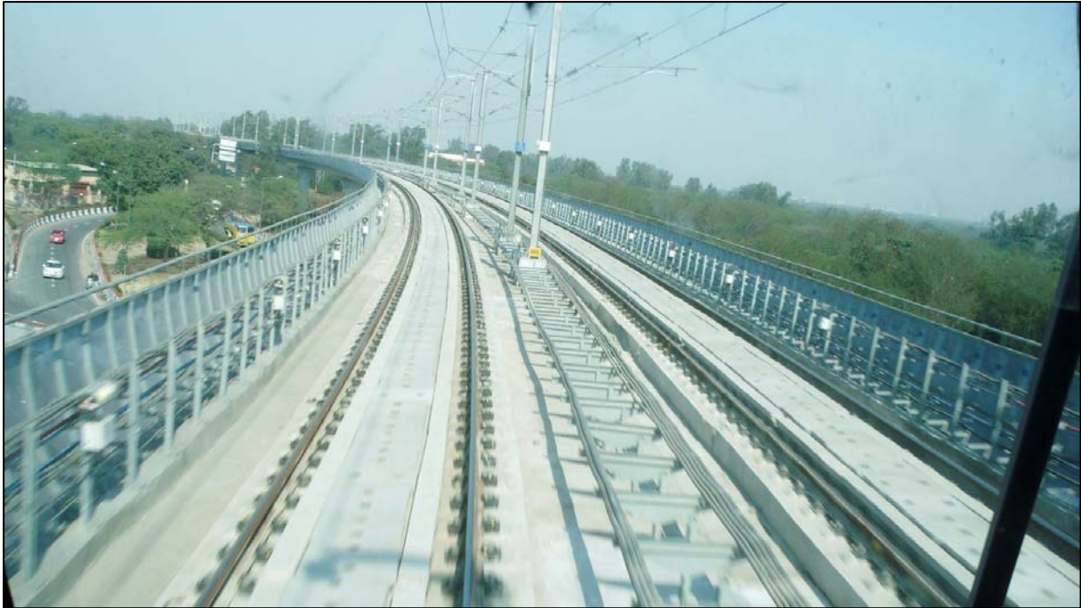
DAMEL Project Double Track on Viaduct during construction phase
