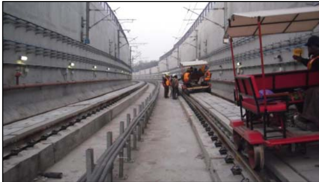
Double Track in Transition Area from Tunnel to Viaduct.
