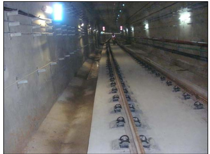
Tunnel Construction Site
