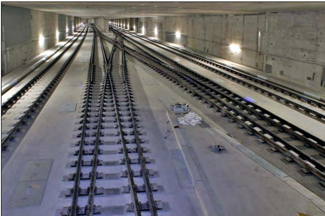
**Track and Turnouts in cut and cover section as floating slab track construction.**
