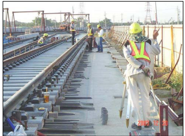
Installation of demo track and turnout
