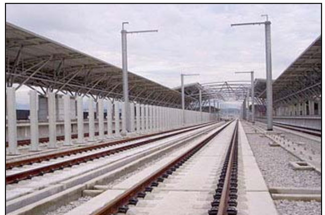
Track work construction was finalised in 1995
