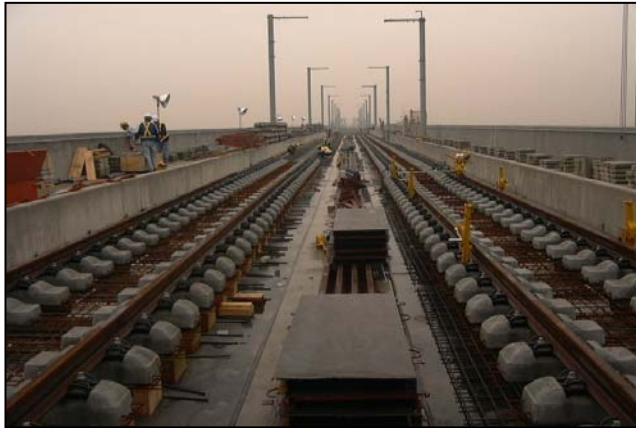
Rheda 2000 Track during construction in station
